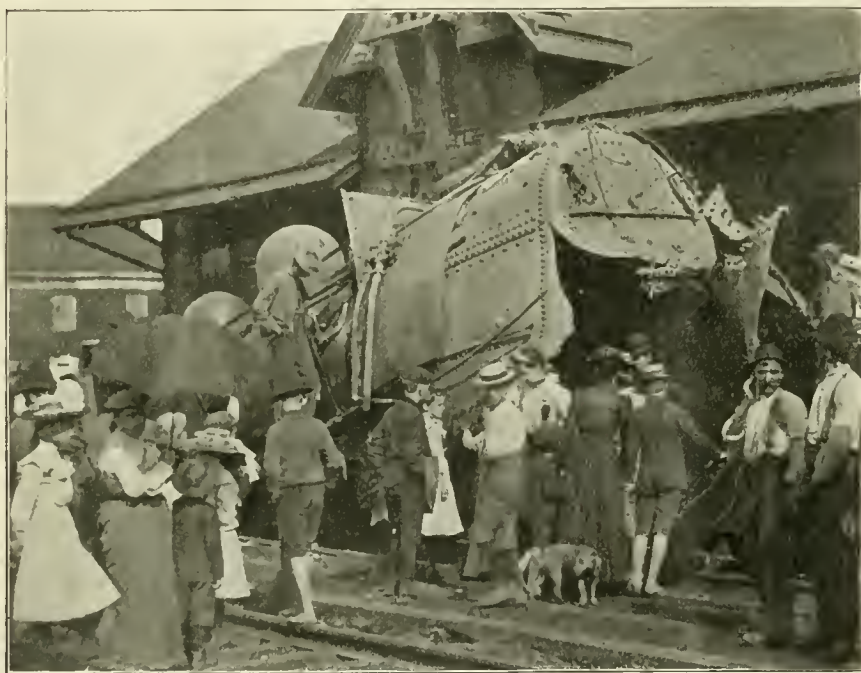
RESULT OF LOCOMOTIVE BOILER EXPLOSION.
